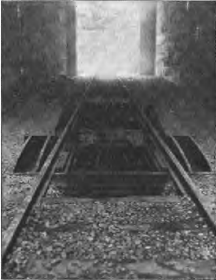
INTERIOR OF CONCRETE EMPLACEMENT FOR 340-MM. FRENCH GUN (LOOKING TOWARD THE ENTRANCE).
